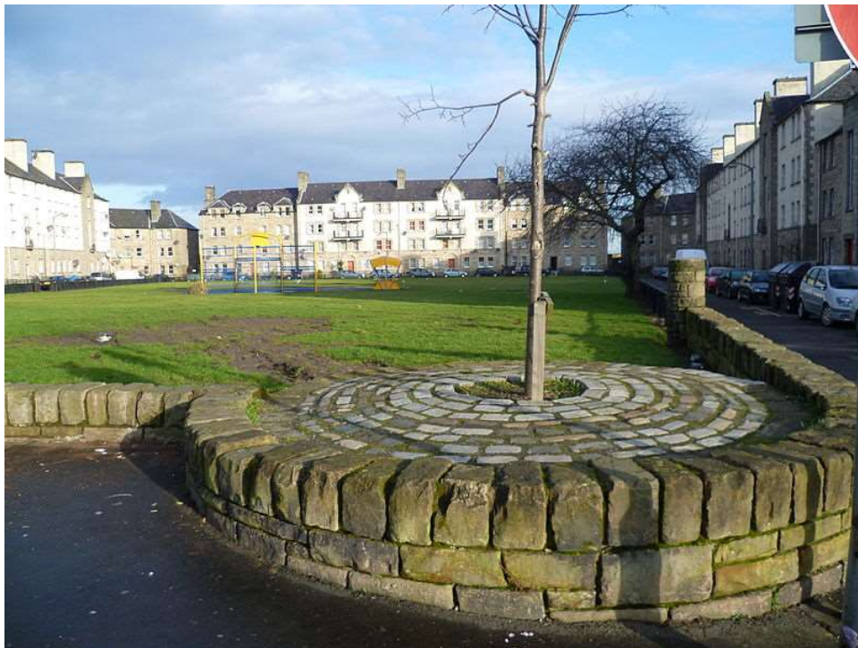
Remains of a barracks wall tower at the north-east corner of Piershill Square West
